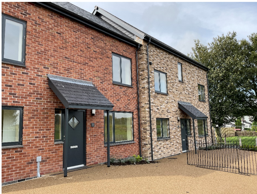
New Council-built homes in Newtown
